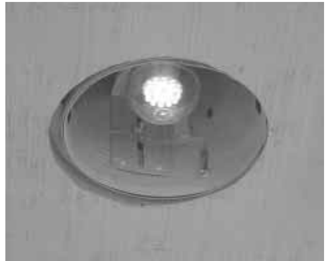
The AC LED—Very efficient, but not quite bright enough for the front porch, and still expensive.
