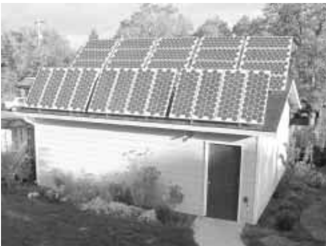
3.2 KW of photovoltaics power the Kerr household.
